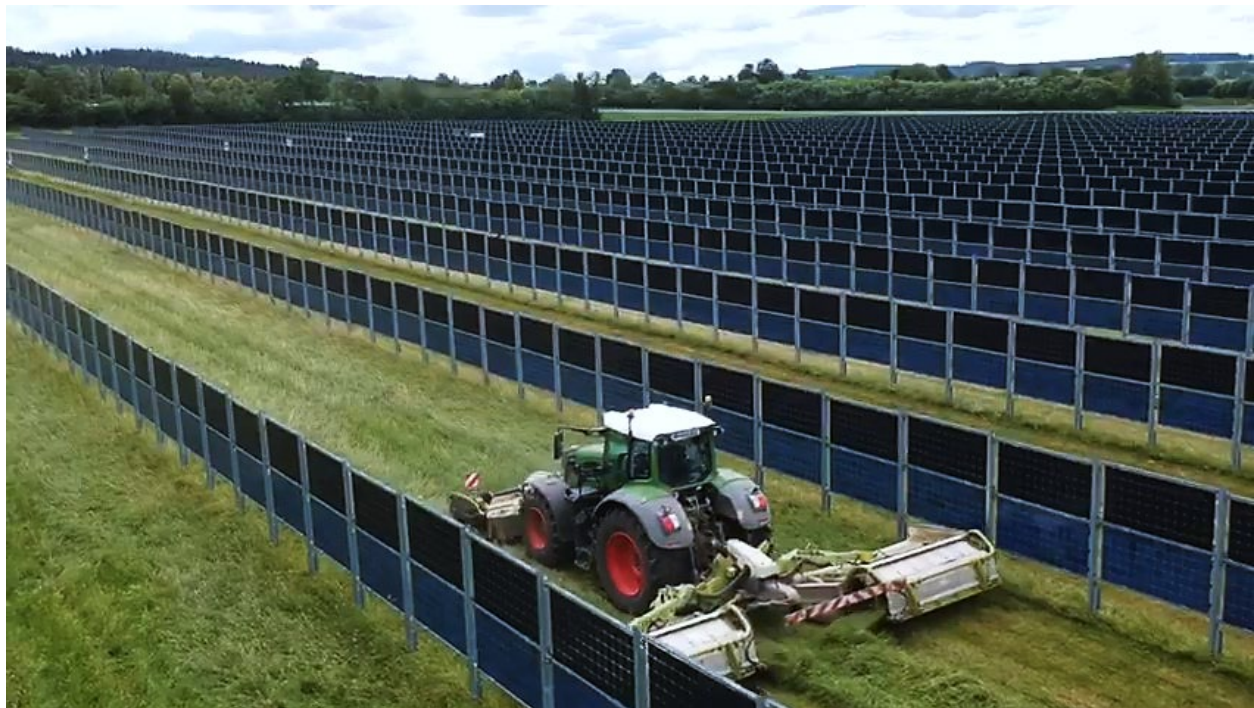
Figure S-8: Bifacial vertically-installed solar panels: Solar Farm, Donauessingen, Germany Photo credit: Next2Sun GmbH, Germany, with permission
