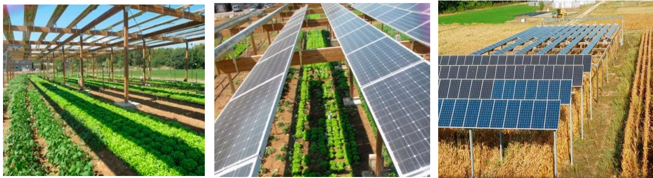
(a) Structure 4 m above the ground (b) Mono-crystalline PV arrays (c) Single-axis sun tracking system
