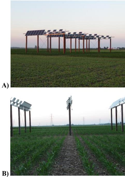
Fig. 1 (a) Image of the ACRE Solar Array taken on 7/8/19 at 9:01PM EST. The planted crop below the array is Maize. Soybeans in the foreground are not a part of this experiment (b) Side view of the ACRE Solar Array taken on 7/8/19 at 9:06 PM showing Maize growth. Size needed adjusting
