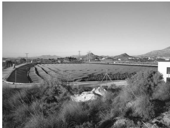
Figure 11: The reservoir completely covered by PV panels.
