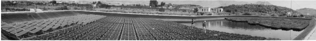
Figure 11: The reservoir completely covered by PV panels.
