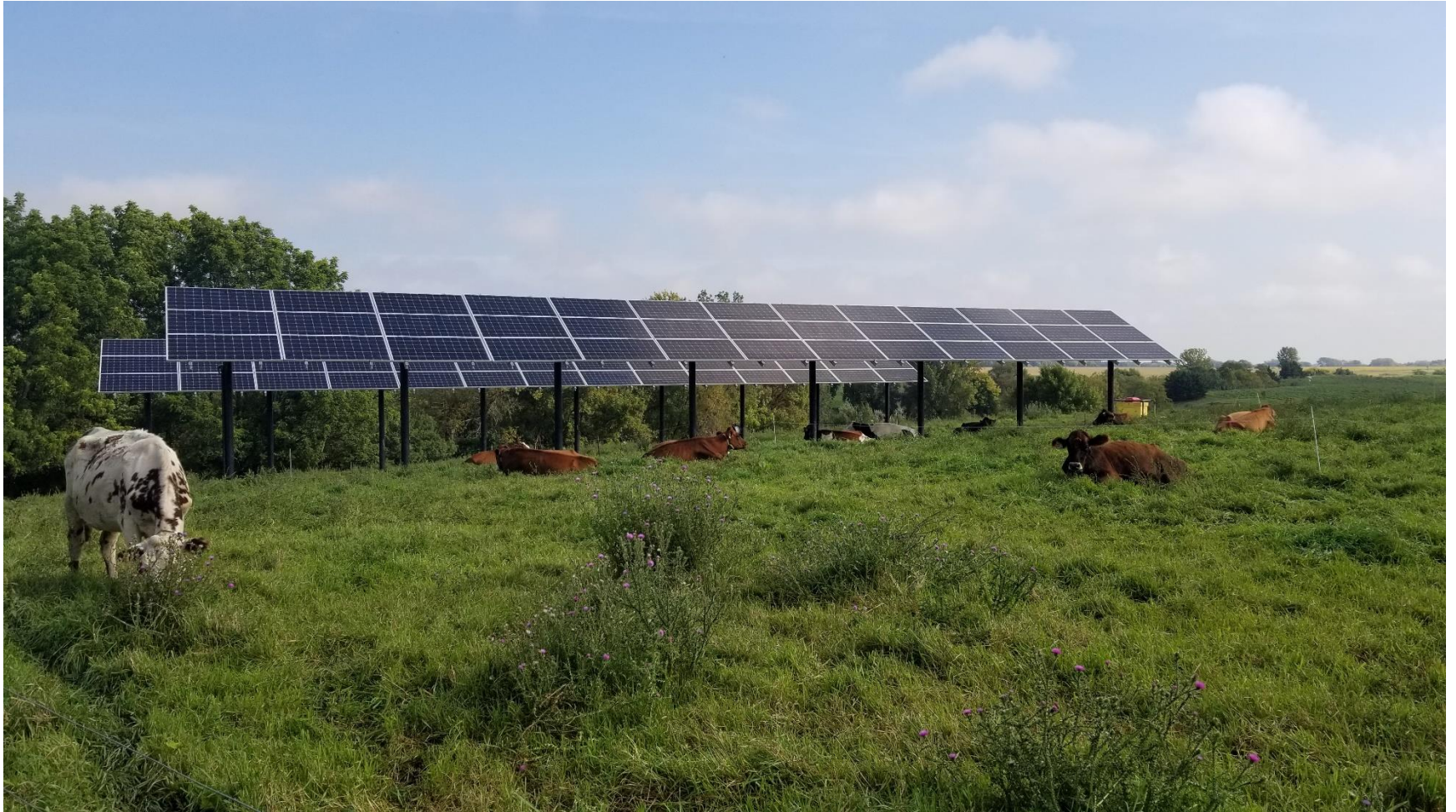
Figure 1. The 30 kilowatt solar photovoltaic ground-mounted system for solar shading at the University of Minnesota West Central Research and Outreach Center in Morris, Minnesota, USA.
