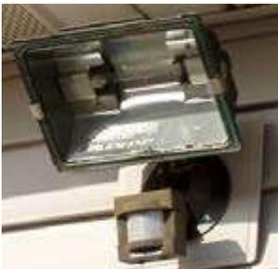
**Figure 7. Halogen yard light with a motion detector.**
