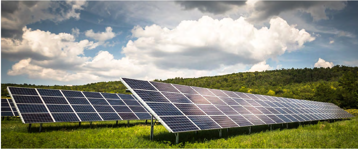
A fixed-tilt solar array, with spacing between rows.
