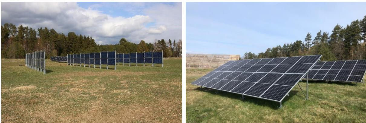
Figure 18 Picture of the vertical system (left) & reference system (right) installed at Kärro Prästgård.
