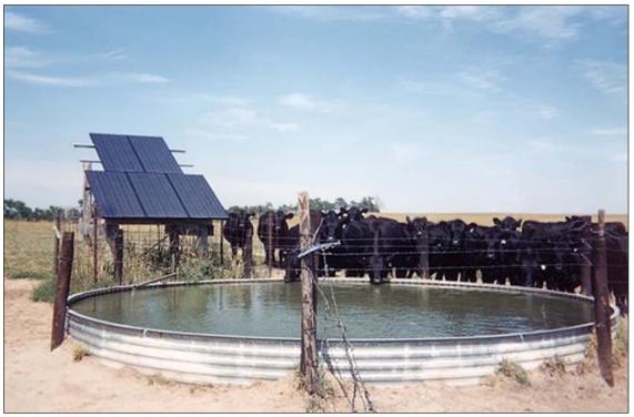
Solar-powered livestock watering system. Photo: NREL
