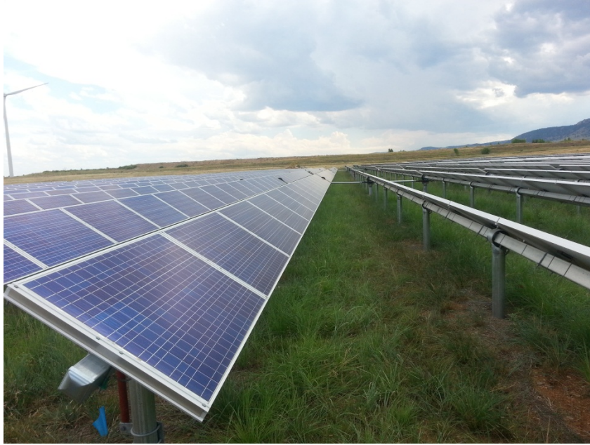
Figure 3. PV panels and vegetation at NREL site. Photo by Jordan Macknick, NREL
