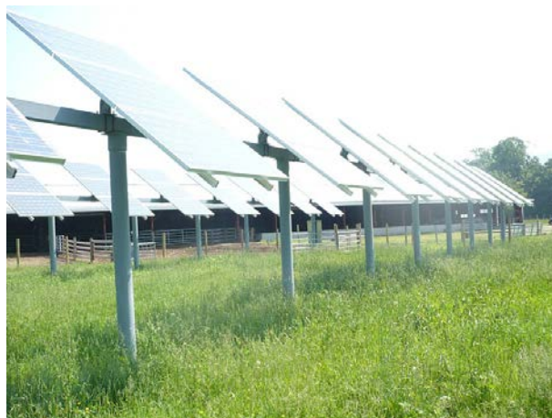
Figure 2. Pasture crops growing under elevated PV panels in Massachusetts. Photo from Stephen Herbert, University of Massachusetts
