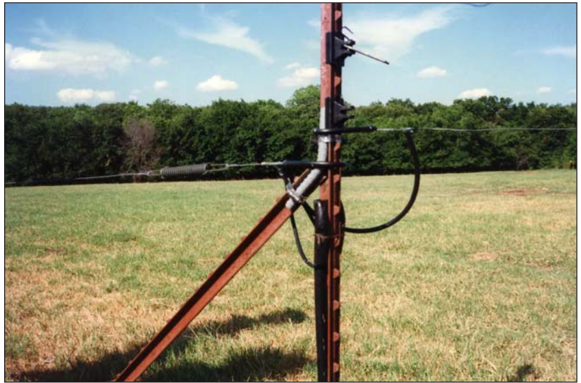
An example of electric fencing using metal T-post. By A. E. Beetz, 2005.
