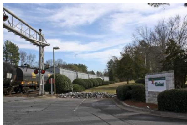
Figure 2: Rail Access at Martin-Marietta, Sodyeco Superfund Site
