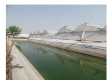
Figure 3. Ponds for rainwater harvesting. They are also being for the conjunctive use of rainwater and groundwater. Copyright: FAO/ Lucie Pluschke near Jaipur, India
