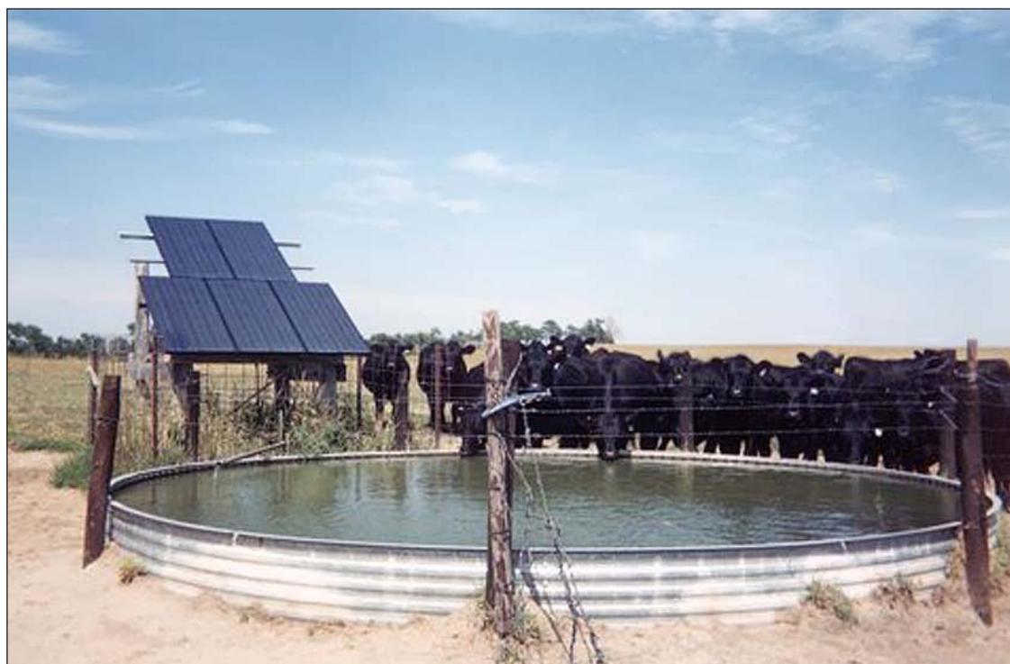
Solar-powered livestock watering system. Photo: NREL
