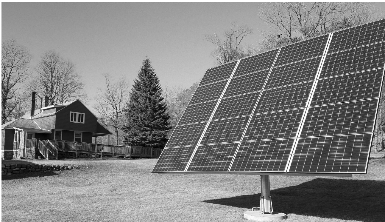
Ground-mounted monopole SES. Photo by Bradley Neumann.
