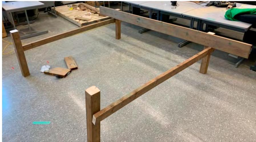
**Figure 2.** The  $2 \times 8$  beam installed between the back posts, with temporary  $2 \times 4$  lateral bracing installed between the left and right posts.
