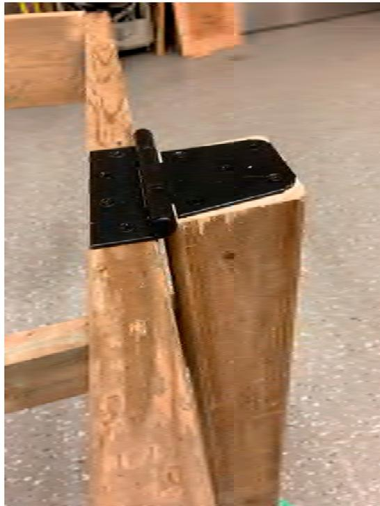
**Figure 4.** Installation of the frame onto the front posts using galvanized gate hinges.
