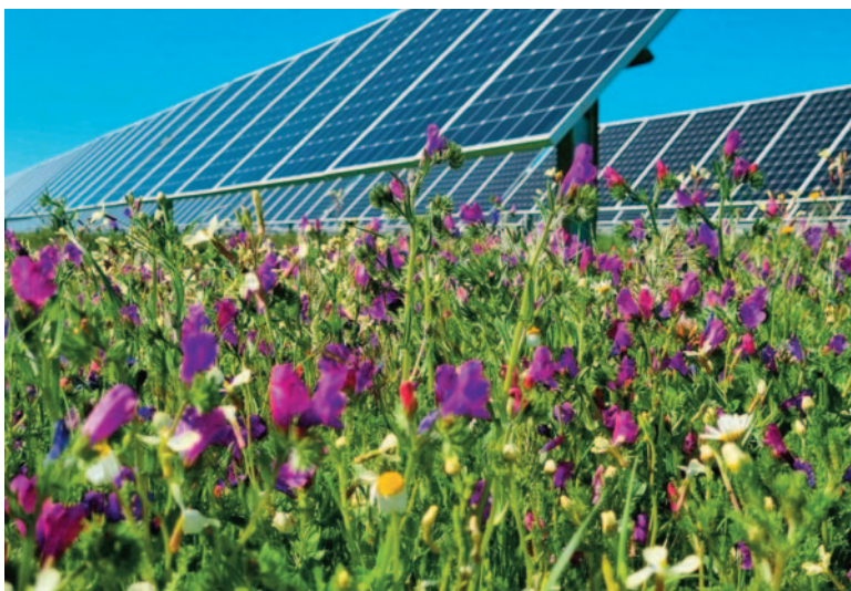
© Enel Green Power.
