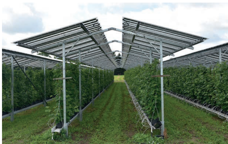
Fig. 38: PV modules with spatially segmented solar cells and protective function in the Netherlands. © BayWa r.e.
