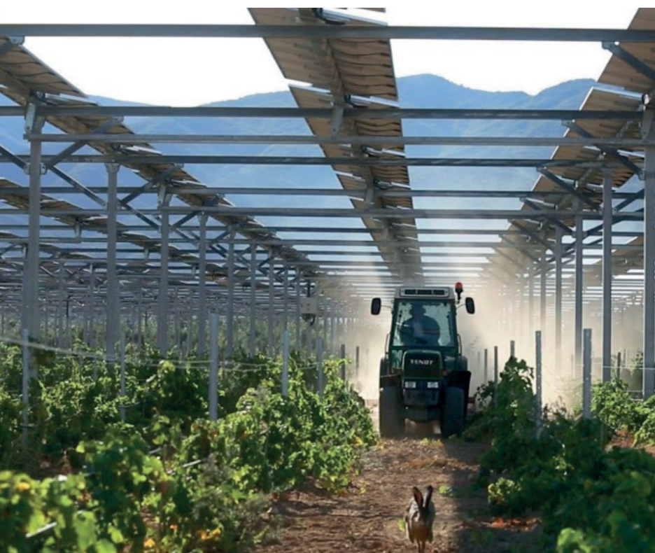
Fig. 44: Overhead system with continuous rows of PV modules. © Sun'Agri
